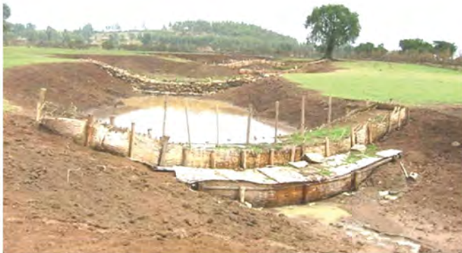
Figure : 20- Brushwood Check dam on field
