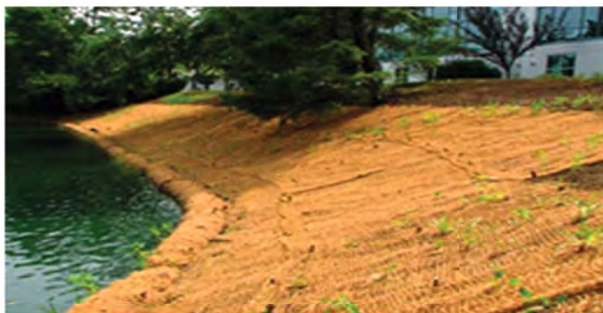
Figure : 18 - Coir Geotextile for Slope stabilization
