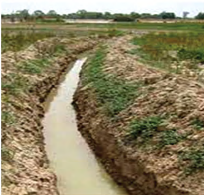
Figure: 21- Construction of Diversion Drain on field
