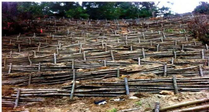
Figure : 17-Contour Wattling as part of Soil Bio- Engineering Measures
