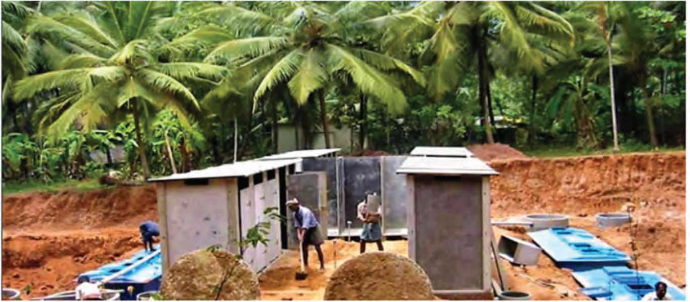
Construction of different toilet blocks connected to two pre-fabricated fibreglass reactor comprising a settling chamber, an aerobic baffled reactor and a final anaerobic filter unit. Source: BORDA (2009)
