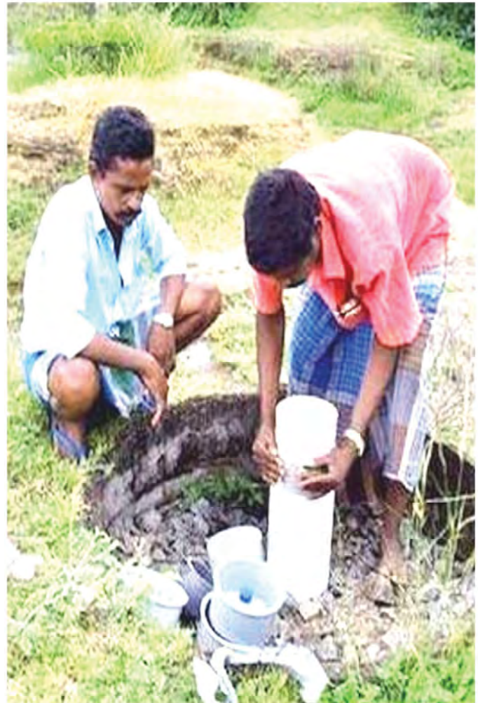
Decommissioning of a defunct/failed borewells
