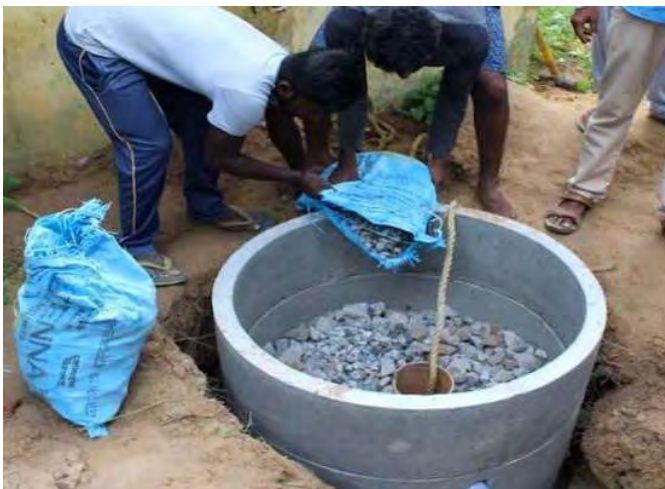
Cement Rings and filtering media around the Defunct bore well utilized for Recharge measures....
